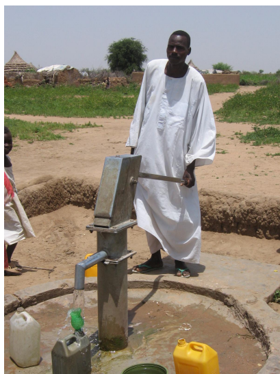
Figure 5. A typical DERO borehole, fitted with an "India" hand-pump. This was installed by SUDO at Um Gozen IDP camp, Mershing.
