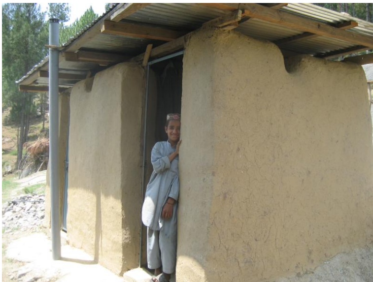
Photo: This double pour flush toilet is also used by family members for showering in the village of Gujar Pata in North-West Frontier Province, Pakistan.
