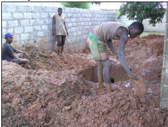
Excavation of pits for the toilets
