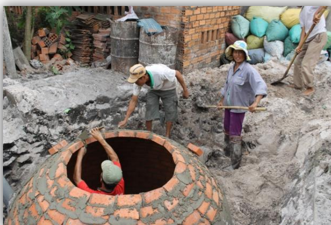
Biogas construction in Quang Tri Province commune in 2012, Photo taken by Le Than Tung, NCA
