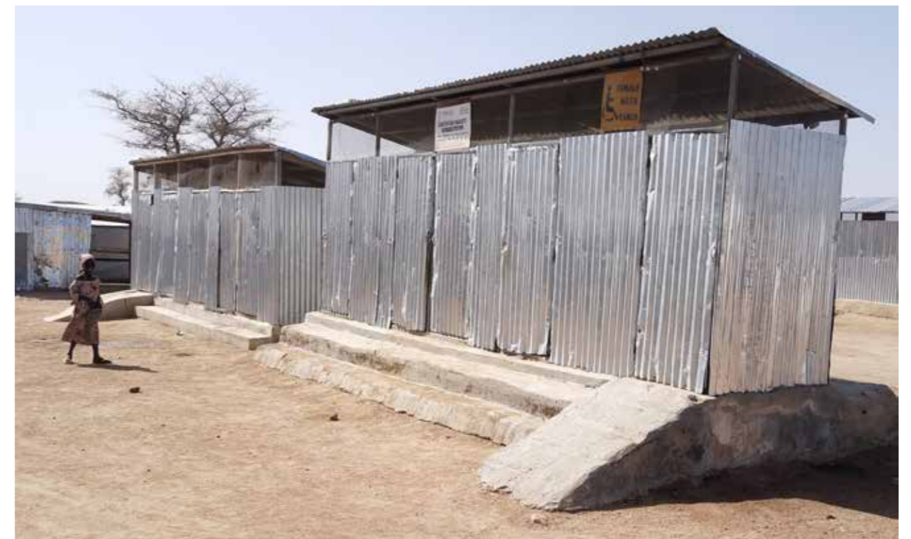
Sanitation facilities enable PWDs access by providing ramps in Pulka IDP camp, Nigeria. Photo: Arthur Laigret/Norwegian Church Aid, Nigeria
