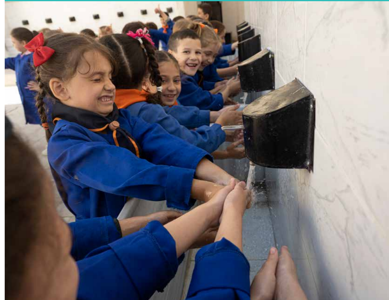
Norwegian Church Aid's partner in Syria has rehabilitated toilets and sinks in schools on the outskirts of Damascus. Photo: Håvard Bjelland/Norwegian Church Aid
