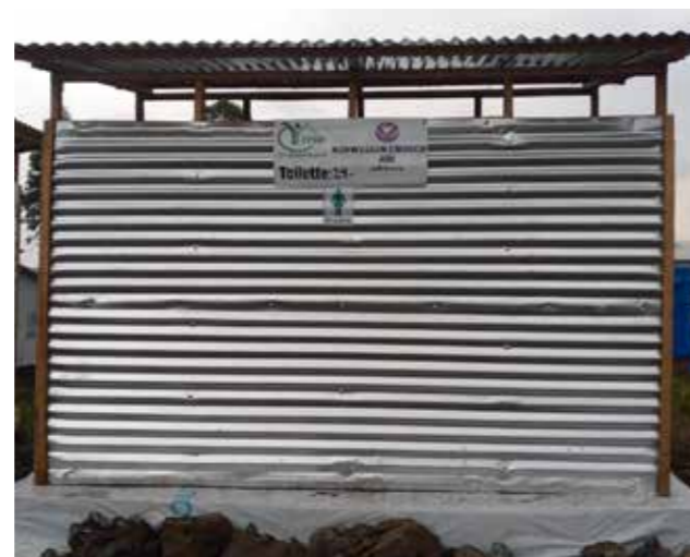
Newly constructed latrines. Photo: Yahona Kadhafi/Norwegian Church Aid, DRC
