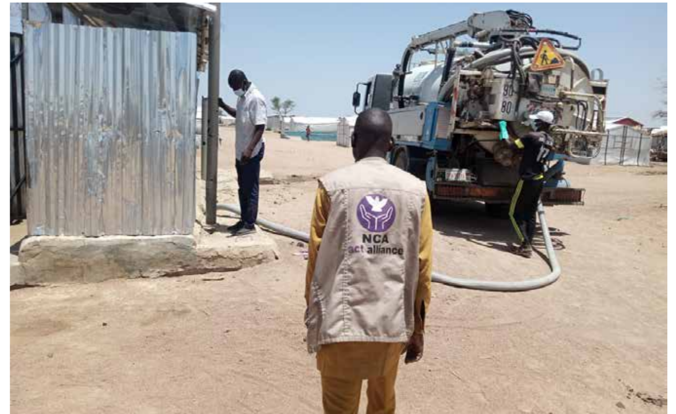
Latrine desludging in Pulka IDP camp. Photo: Arthur Laigret/Norwegian Church Aid, Nigeria
