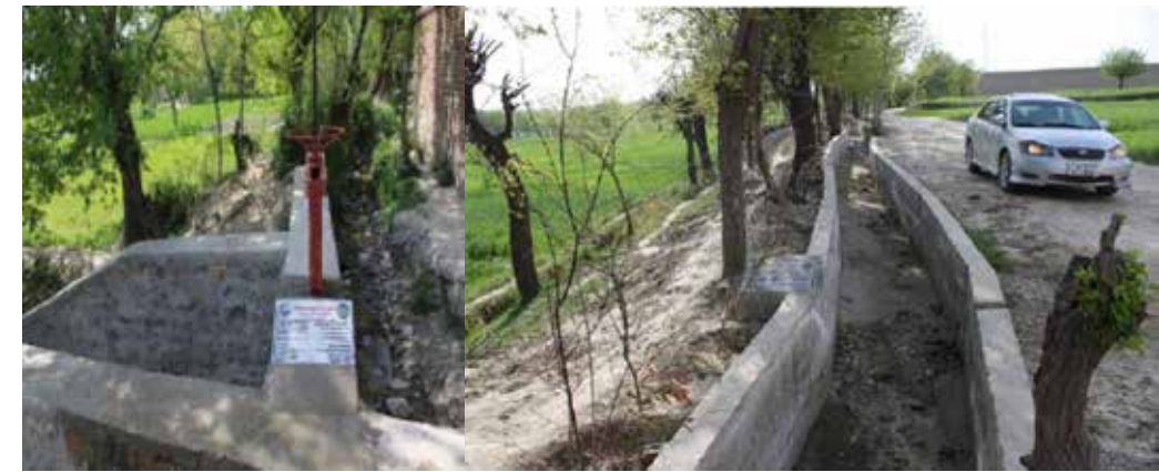
Water Canal and division box for irrigation management in Khost province, Afghanistan, built by NCA in 2021. Photo: Afghan Development Association (ADA)
