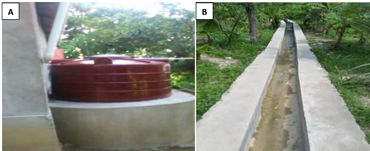
Figure 3 : Examples of sustainable interventions A) Family water tank in Floquette, Petit Goâve and B) Irrigation canal at Arnoux, Petit Goâve
