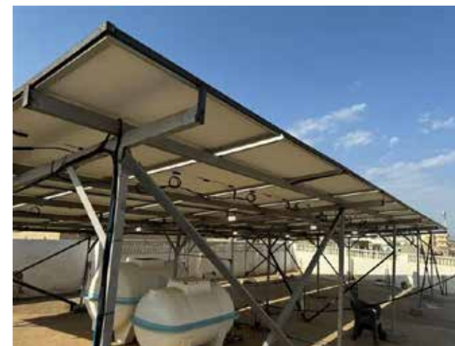
Installed 36 PV panels and 240 kWh capacity Lithium battery-pack at the Port Sudan office in Sudan. Photo: Norwegian Church Aid, Sudan
