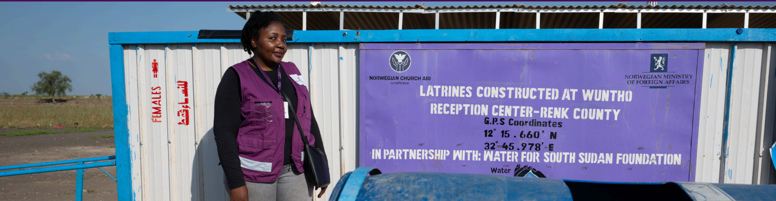
WASH Manager Cynthia Gwisai at installed toilets and showers. Photo: Håvard Bjelland/Norwegian Church Aid
